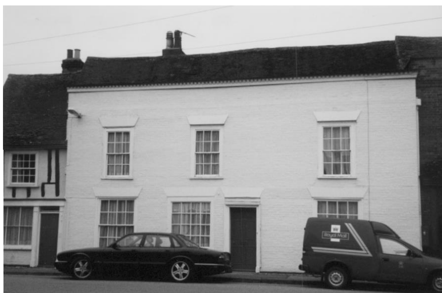
8c. The former Vine Public House, 1999
