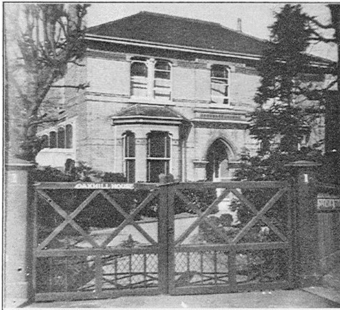
27a. Oakhill House, No.1 Oakhill, Putney
